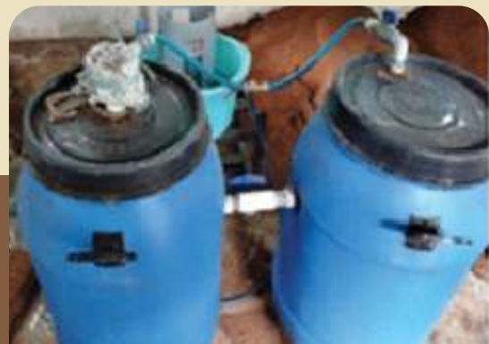
Anaerobic Fermenter for the biological treatment of Ret liquor
