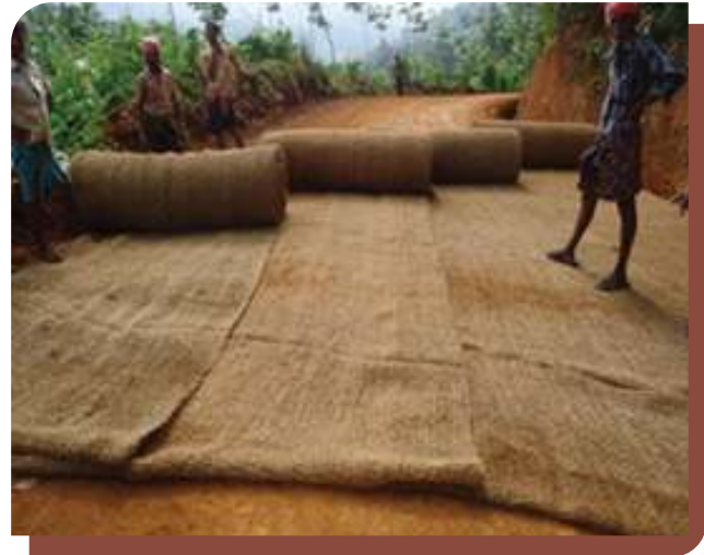
Fig. 4 Laying of Coir Geotextile
