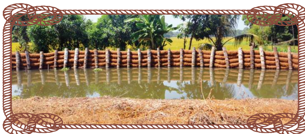
Canal bank protected by cocolog
